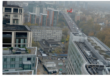
Helicopter flies one of the two Carrier replacement chillers into position.
