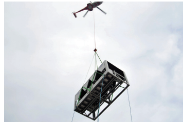
Helicopter with chiller and trailing grab lines for stability.
