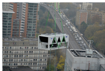
Chiller airborne slung beneath the helicopter.
